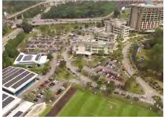
An aerial view of the solar PV system installed at Persada PLUS.
