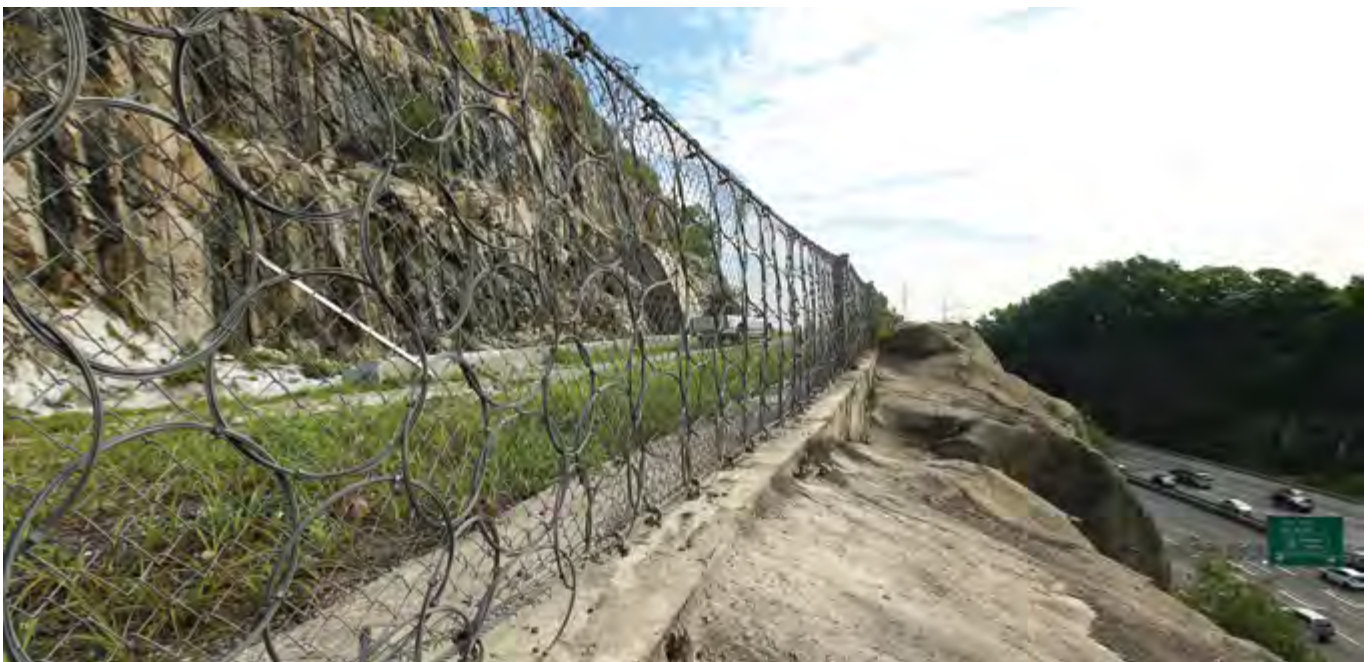
Our rock-fall barrier, along the New Klang Valley Expressway (NKVE).
