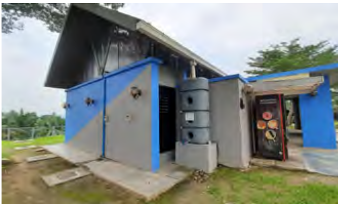
Our rainwater harvesting systems at Lay-by Yong Peng.
