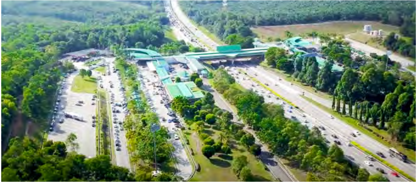
An aerial view of Overhead Bridge Restaurant (OBR) Ayer Keroh.
