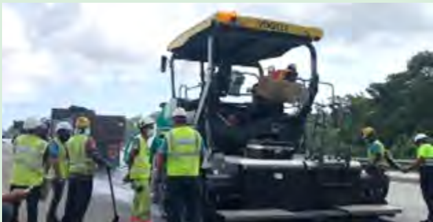
The trial lay location for HIP recycled asphalt at Section C3.
