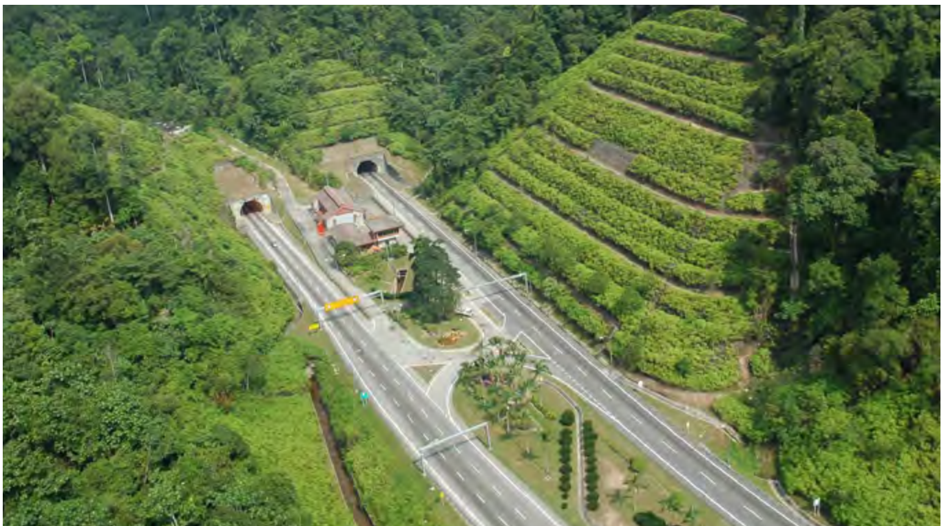
An aerial view of the Menora Tunnel and Meru Tunnel, along the North-South Expressway (NSE).
